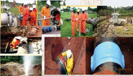
Intelligent Pigging, Cathodic Protection and On-line Leak Repairs Operation
