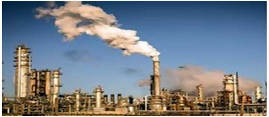
Fig. 1: Oil, Gas and Petrochemical Plant, Port-Harcourt, Nigeria
